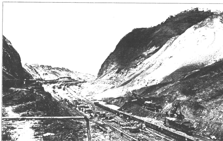
Culebra cut on January 4, 1913, just after a land slide. Note huge track-mounted steam shovels at the right. ("The Panama Gateway," Joseph Bucklin Bishop, 1913)
