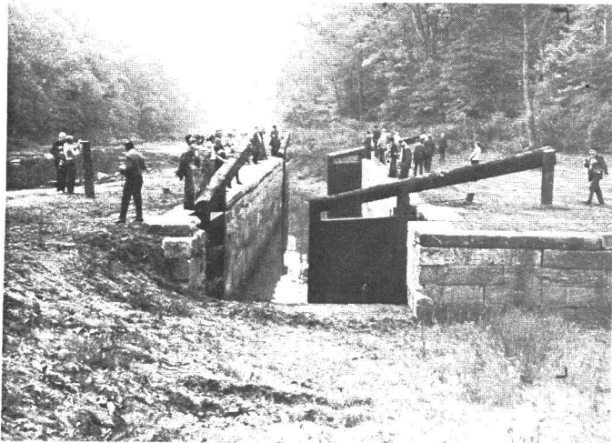
Lock Number 50 on the eastern section of the Sandy and Beaver Canal, near the canal town of Frederickstown, Ohio, has been dug out of the mud and completely restored, with mitre-gates which work. (Photo by the Author.)
