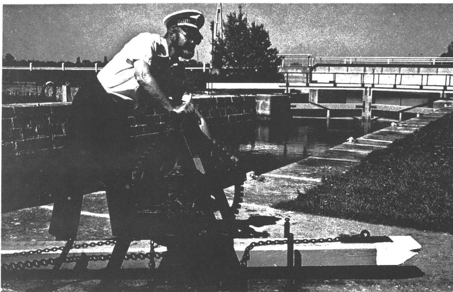
Rideau Canal lock gates are assisted by a hand-operated chain and winch. (Parks Canada photo.)
